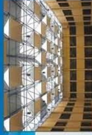
Public Administration Institute Dammam
