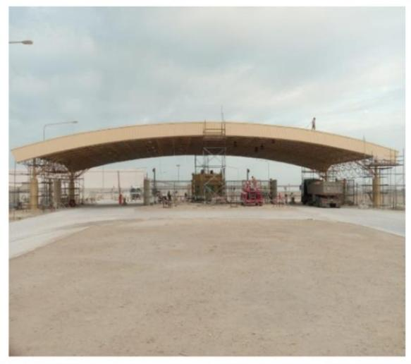
No other space frame system in the market is known to possess such degree of self-attenuation or gap-bridging capability at the face of high load and long span applications inherently characterized by the ME-SSP system. Absorb the lateral displacements of the support bases by the flexure moment capability of the support shaft.
